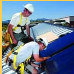
Students of Univ. of Colorado mount solar panels on their home's roof Photo: Solar Decathlon
